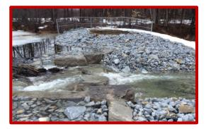
Good News....the initial stage of our Spring freshet is outflowing rapidly and without any real resistance down the outlet. There is a small amount of wood debris (short logs/branches) that has collected over the winter at the leading edge of spillway which will be removed once overall site is fully accessible. Association volunteers will be assisting the Township, as to ensure unobstructed outflow of any high level spring water levels.
