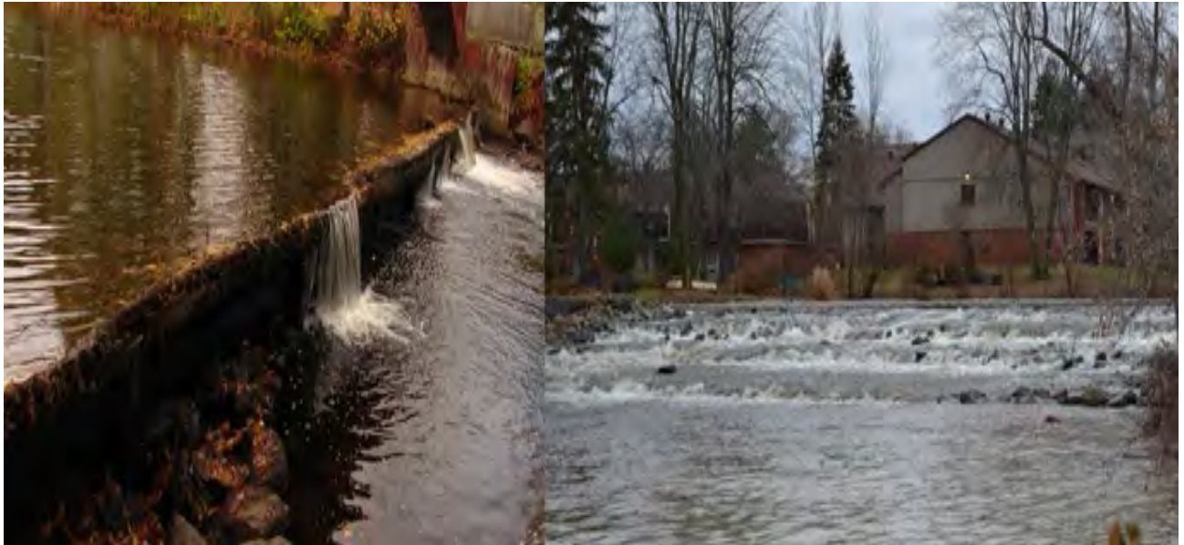
Figure 4-1. Before and after conversion of a traditional structural (wooden) weir to a rocky ramp
